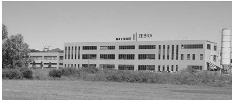
Fig. 17. New ZEBRA battery factory on the MES-DEA site in Stabio, Switzerland.
